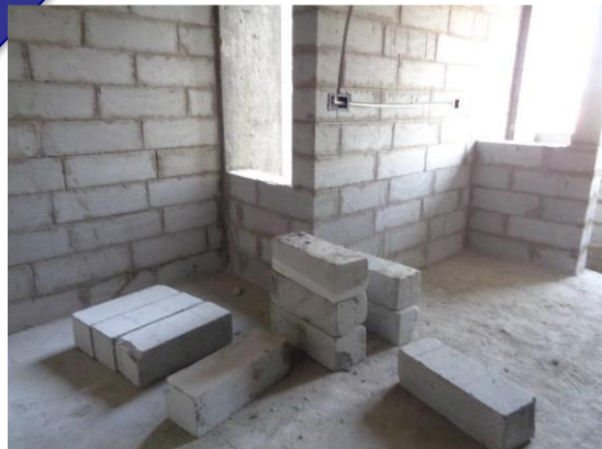
200 mm AAC block with U value – 0.7 w/m 2 k
