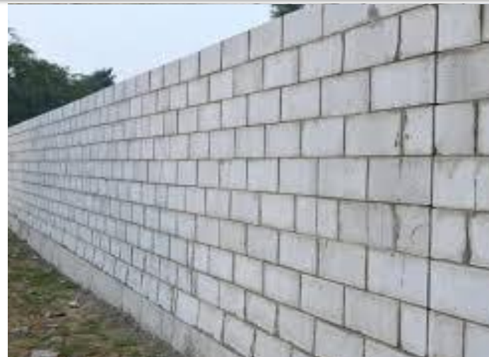
200 mm Solid Concrete Block with 15 mm plaster on both sides – U Value 2.8 \text{ W/m}^2\text{K}
