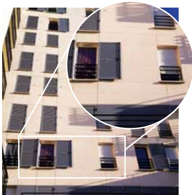
Figure 4.7b Hinged shutters and top rolling shutters
