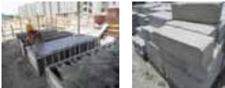
CLC blocks produced on-site
