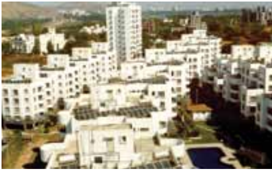
Figure 8.4 Solar water heater systems installed on rooftop
