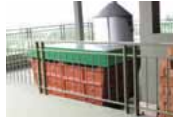
On-site waste management
