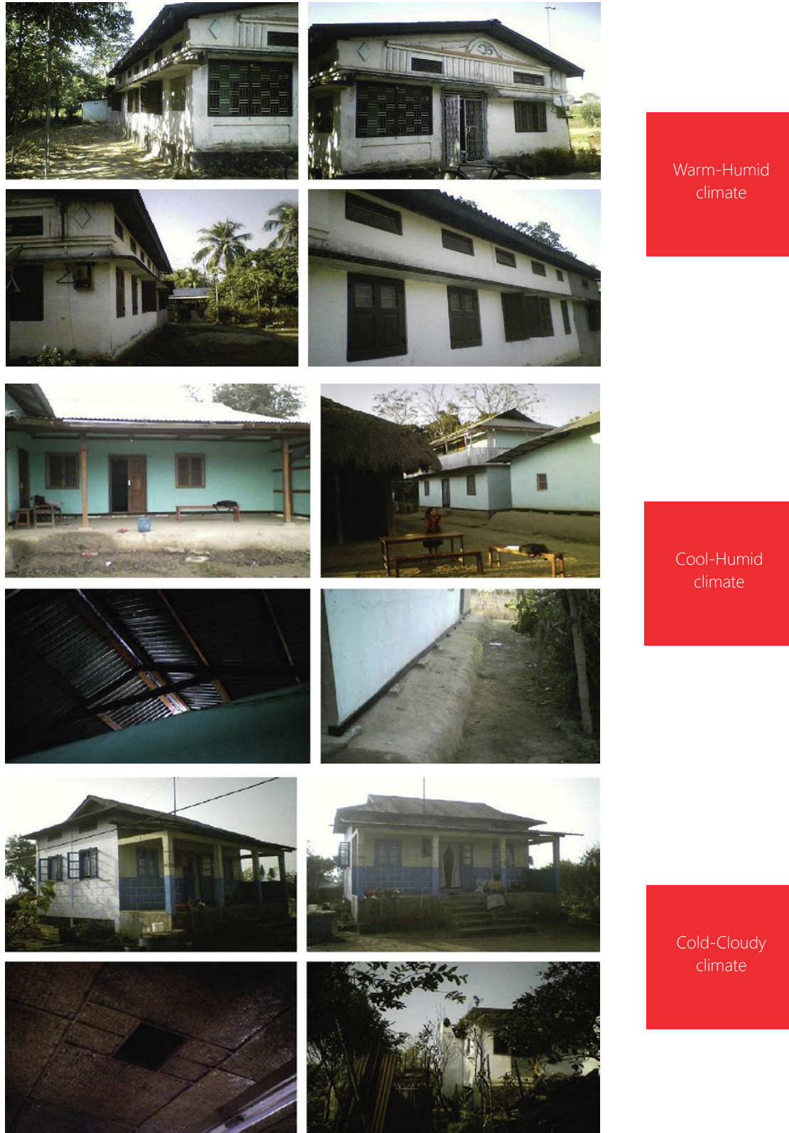
Figure 127: Photographs of vernacular houses selected for long-term monitoring
