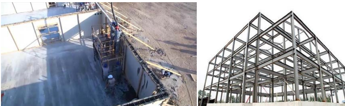
Figure 105: On-site construction using PVC Stay-in-place formwork system. Source: (MoHUA. GoI, 2021)
